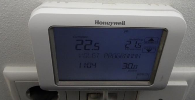
Controlling air-water heatpump
