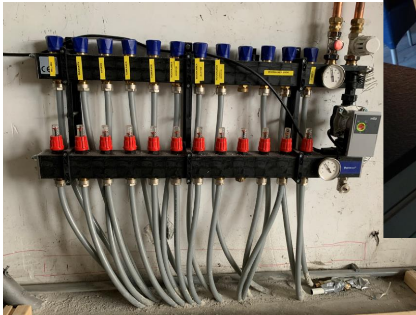
Low temperature floor heating system
